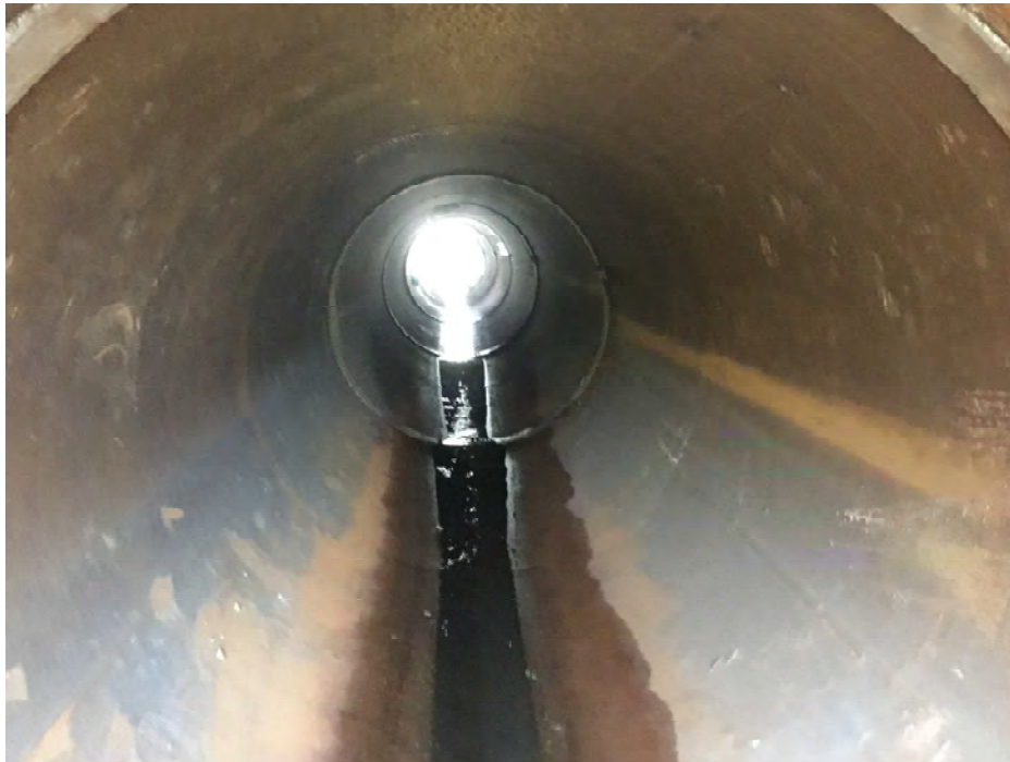
PHOTO 5 Condition Description Looking West through culvert
