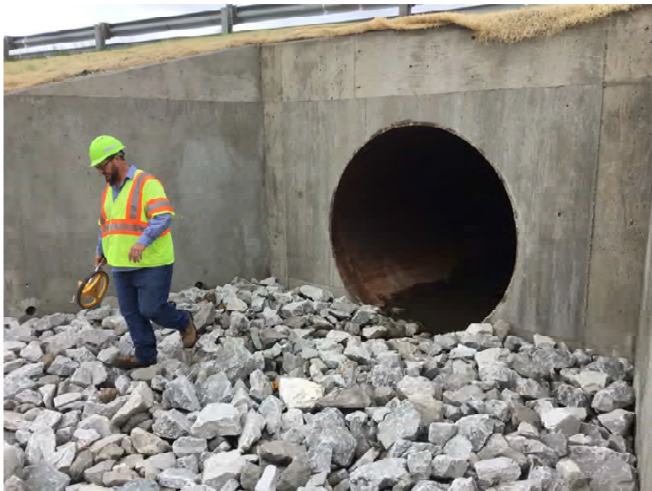
PHOTO 4 Elevation, Condition Description Profile looking East
