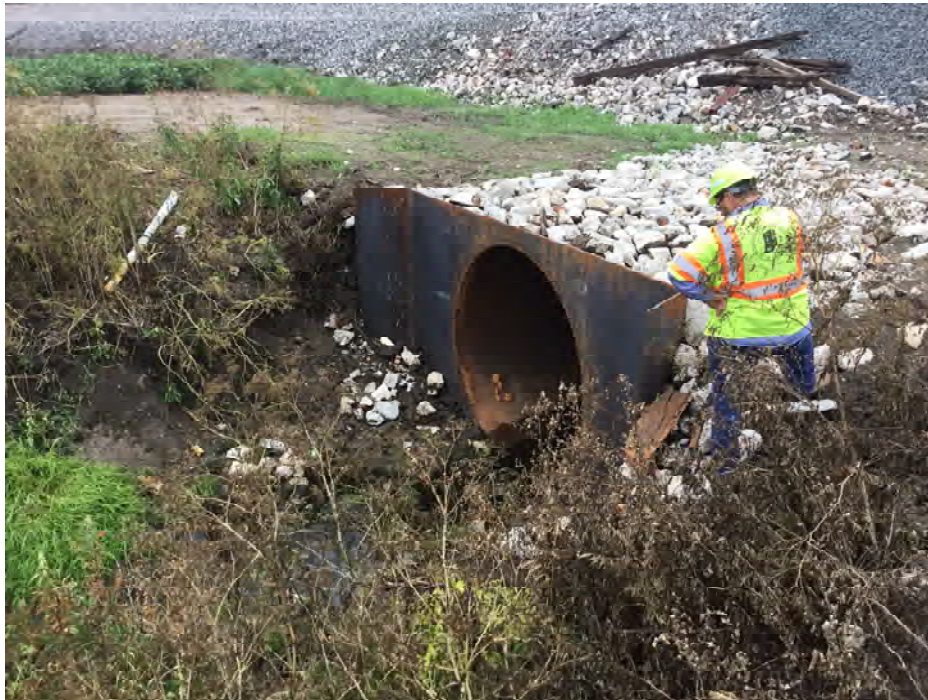
PHOTO 3 Elevation, Condition Description Profile looking West
