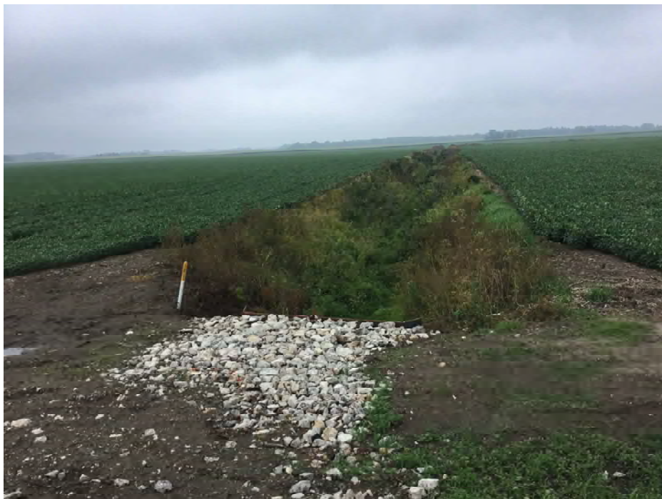
PHOTO 6 Condition Description Channel alignment on East side of road
