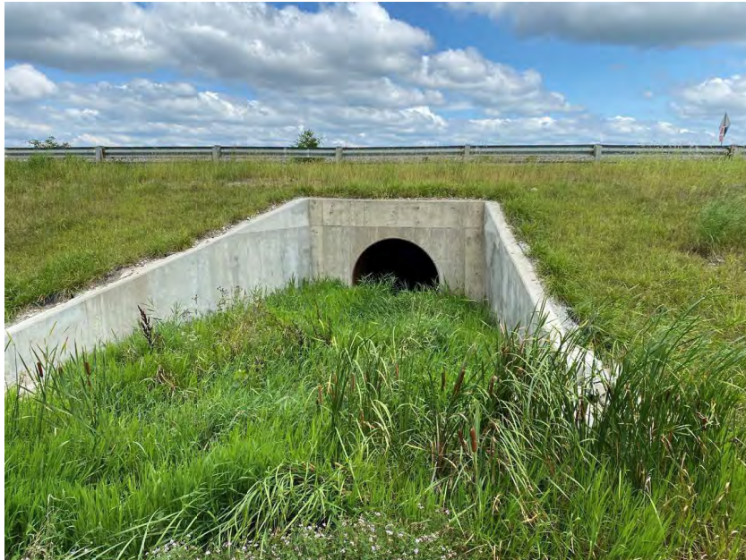
Photo 47. Taken west of US 231 facing east showing Wetland D.
