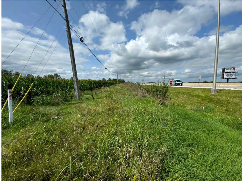
Photo 13. Taken west of US 231 showing roadside vegetation and surrounding area.
