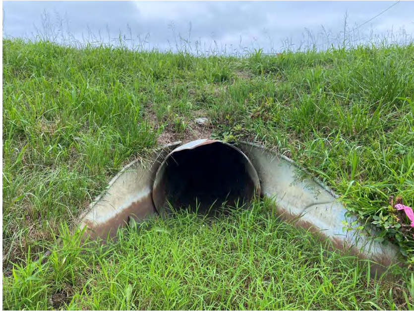
Photo 1. Taken east of US 231 facing north showing the pipe (inlet) underneath the subject drive.
