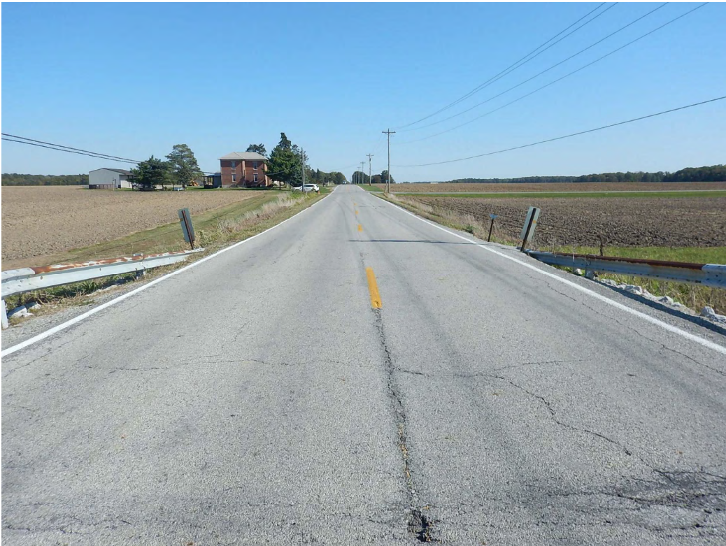
6. From Bridge 277 looking east at the bridge approach and Monroeville Road.
