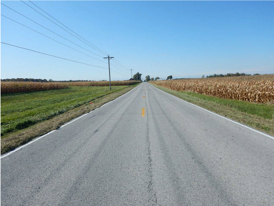
13. From the middle of Monroeville Road (western side of project area) looking west at Monroeville Road and western project area terminus.
