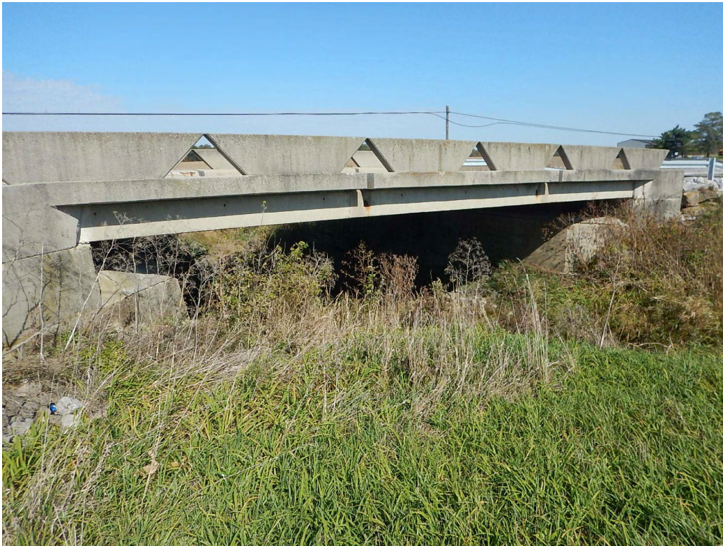
1. From the south side of Monroeville Road looking northeast at Bridge 277.
