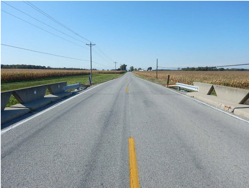
9. From Bridge 277 looking west at the bridge approach and Monroeville Road.
