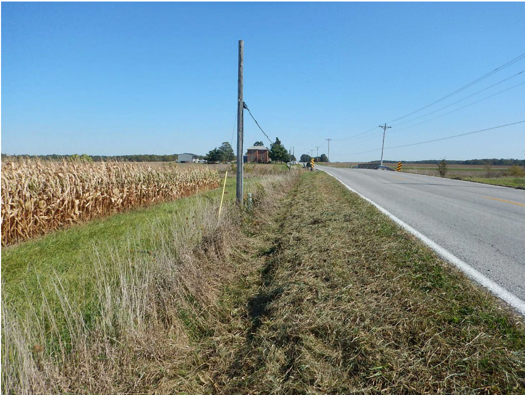
12. From the north side of Monroeville Road (western side of project area) looking east at the Monroeville Road and surrounding landscape (Bridge 277 in distance).
