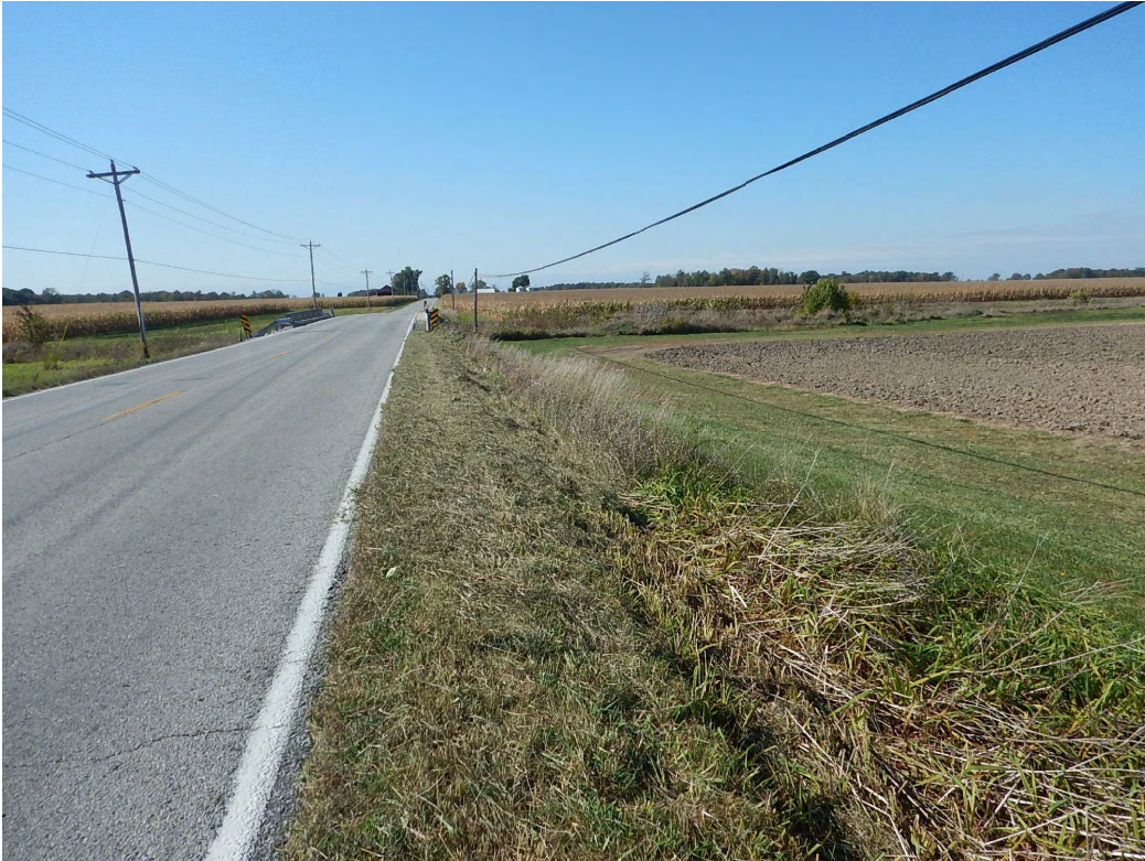
5. From the north side of Monroeville Road (eastern side of project area) looking west at the Monroeville Road and surrounding landscape (Bridge 277 in distance).
